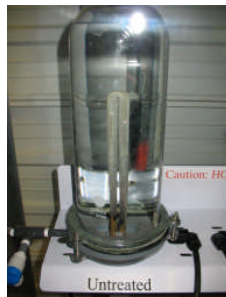
Scale Build-Up (With untreated water.)
